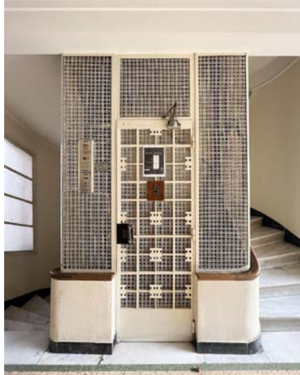
athens_mon_amour The elevator shaft in the prominent Savvidis building on Plateia Agyptou, designed by Nikolaos Nikolaidis in 1934, renowned Greek architect of the interwar period in Athens 🇬🇷
