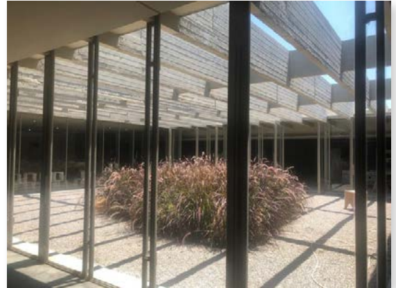
The Guest House at the RKIF rehabilitated to become Minjara Platform by Maya Hmeidan-UNESCO Beirut
